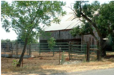
Example of acceptable corrals.
